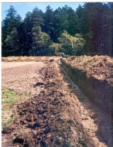
Drain Tiling Upper Field (See Hydrology Map In Appendix)
